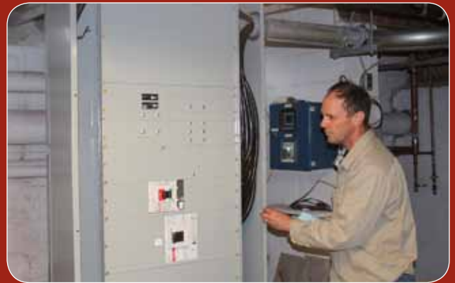
An electrician works to upgrade the systems in St. Joseph's Hall.
